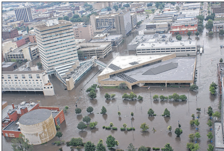
The former Downtown Library building of the Cedar Rapids Public Library is seen from an aerial view after the flood of June 2008 inundated downtown Cedar Rapids. The library lost 160,000 books and media items from the flood, which forced the building to be gutted. (Cedar Rapids Public Library)
