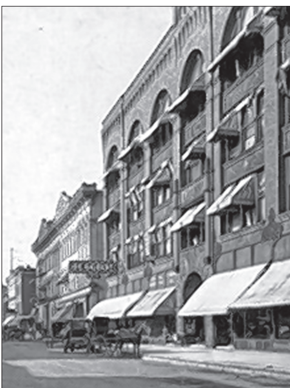
In 1897, the first Cedar Rapids Public Library was outfitted in a room in the Granby Building at the corner of Third Avenue and Second Street SE. (Cedar Rapids Public Library)
