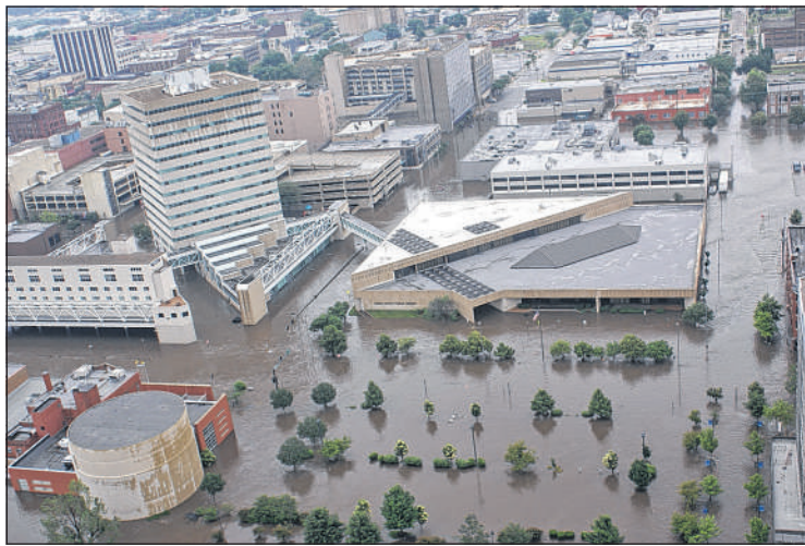
The former Downtown Library building of the Cedar Rapids Public Library is seen from an aerial view after the flood of June 2008 inundated downtown Cedar Rapids. The library lost 160,000 books and media items from the flood, which forced the building to be gutted. (Cedar Rapids Public Library)
