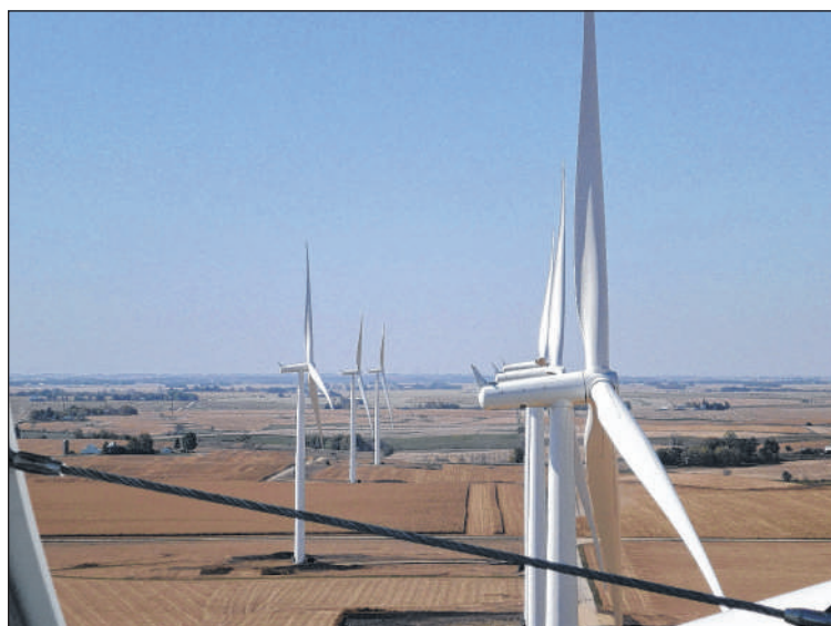
A view of MidAmerican Energy's Vienna wind project in Tama and Marshall counties from atop the nacelle of one of the wind turbines is shown in an undated photo. (MidAmerican Energy)
