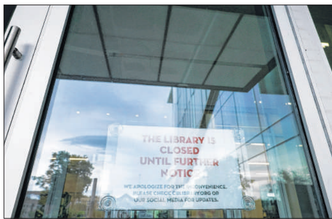
The downtown Cedar Rapids Public Library remains closed Wednesday as cleanup continues after a fire July 27 in a light fixture. (Jim Slosiarek/The Gazette)
